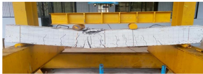
Fig 3.1 Cracking pattern of control beam
