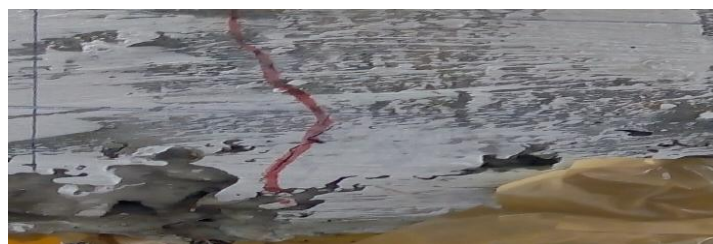
Fig 3.3 First Crack of SFRC Beam
