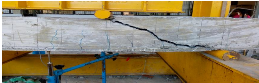
Fig 3.6 Cracking Pattern of EFRc Beam
