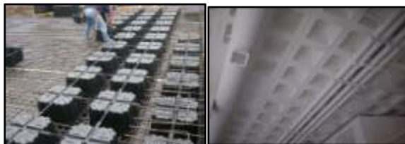
Fig 10. During construction Fig 11. After construction
