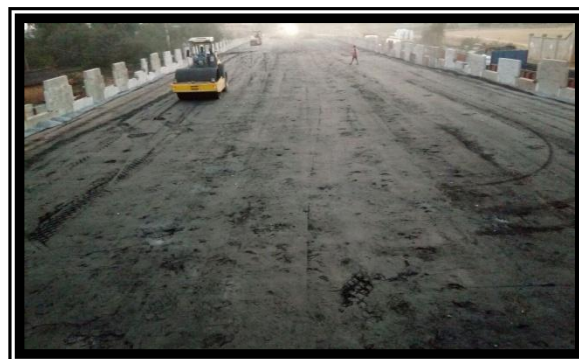
Fig.6.Pond ash rolling at Rewall back filling.
