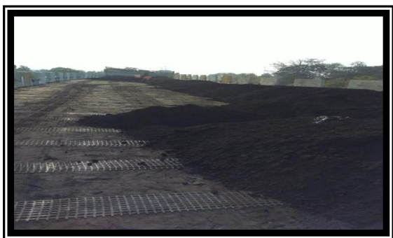
Fig.4.Pond ash dumping at Rewall
