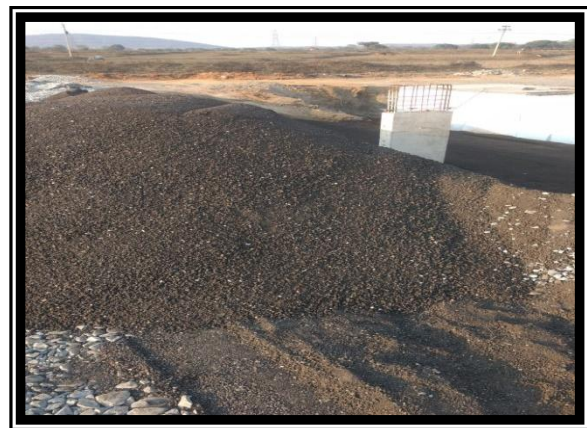
Fig.9. Slag used in structure back filling
