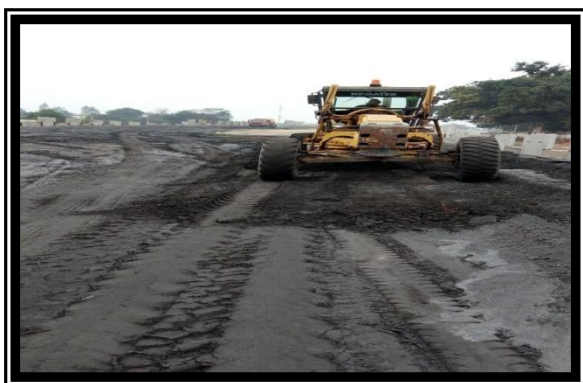
Fig.5.Pond ash spreading with Grader
