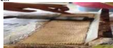
Fig.9. Applying roller on the laminate to remove entrapped air.
