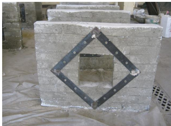
Figure (12): Details of the used rehabilitation technique using (3x50 mm) diagonal steel plate around opening at both sides.
