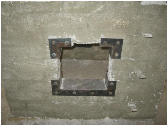
Figure (9): Details of the used rehabilitation technique using (2x40mm) L&U-shaped steel plate inside opening corners welded with U & L-shaped steel plate.
