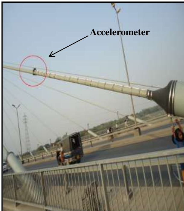
Fig. 4.1 Accelerometer on the Cable
