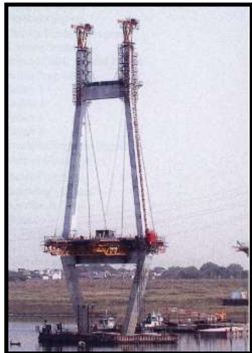
Fig. 3.1 Pylon at Construction Time
