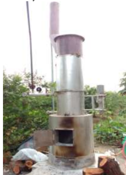
Fig4. Modified Boiler With Chimney
