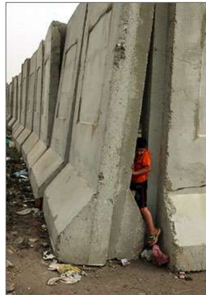
Fig. 13: Baghdad: The negative impact of the concrete walls. [3]
