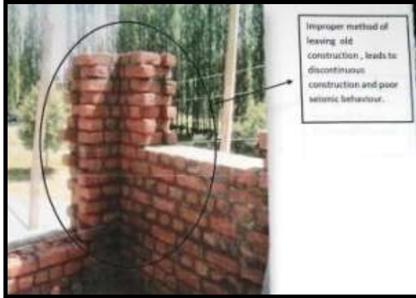
FIG C Construction of the corner joint
