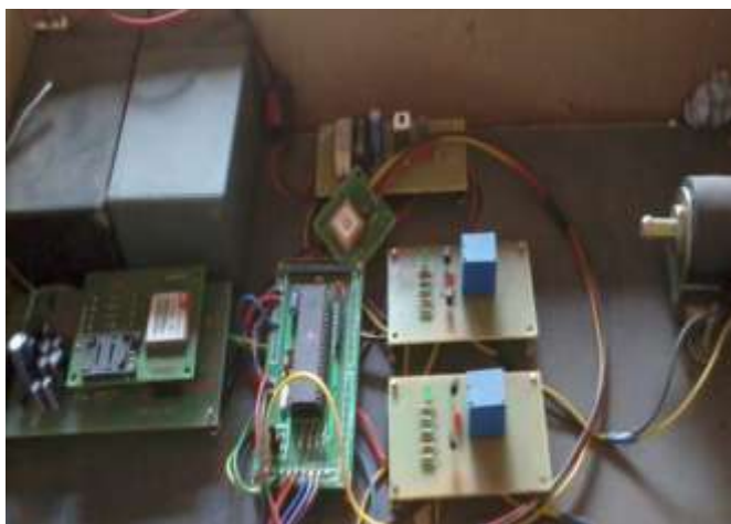
Fig 5. GSM and GPS interfaced with microcontroller and solenoid valves connected with driver relay circuit.
