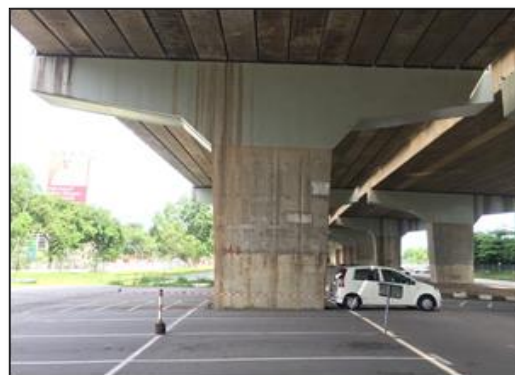
Fig. 1 Crosshead of the Bridge
