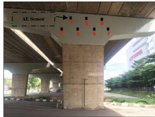
Fig. 3 AE Sensor layout at crosshead
