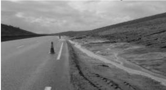
Fig 2 : Tangier-Port highway (mileage point 40 towards the Port)
