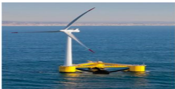
Figure: WindWaveFloat, a floating hybrid wave-wind device (courtesy of Wikimedia [5])
