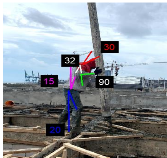
Fig. 4 Posture at the pouring work
