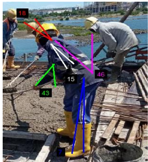
Fig. 5 Posture at the stages of levelling work
