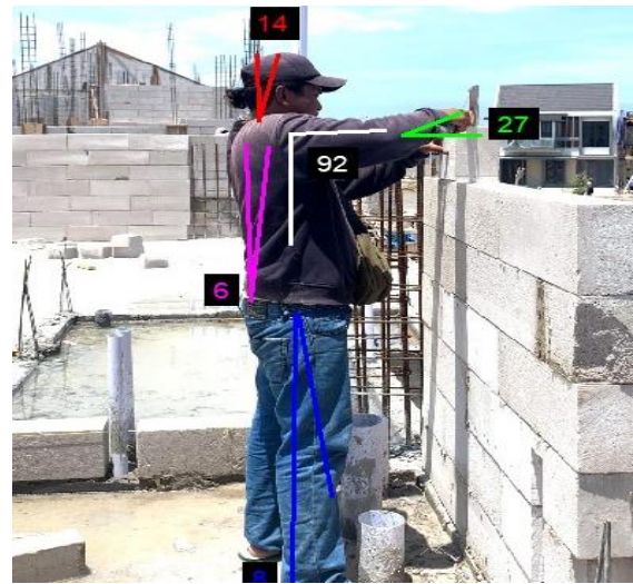
Fig. 7 Posture at the stages of laying light brick
