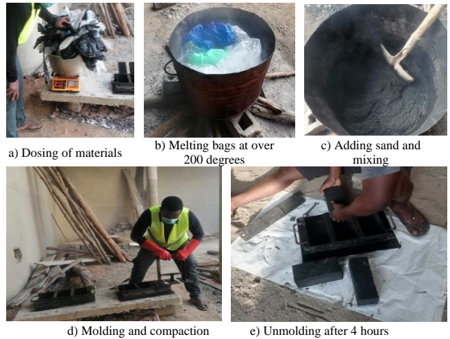
Fig. 4 Pavers making process
