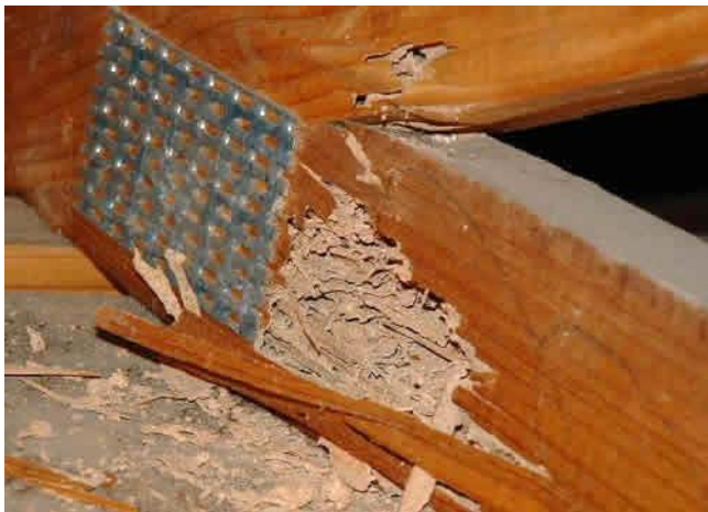
Fig. 2 Termite attack
