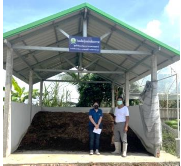
Fig. 3 The composting plant with palm waste material
