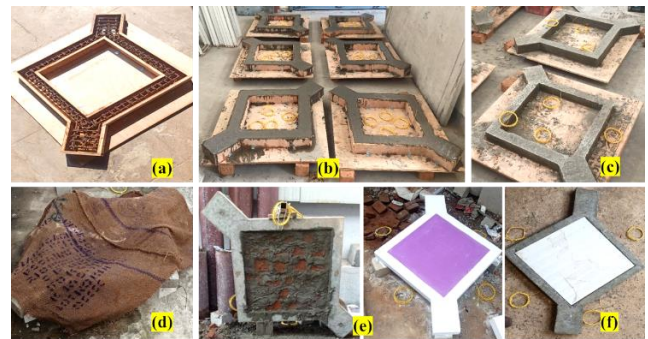
Fig. 11 Preparation of RC frames (a) Mould with reinforcement (b) Casting of frames (c) Demoulding (d) Curing (e) Masonry infilled frame (f) Sandwich infilled frame
