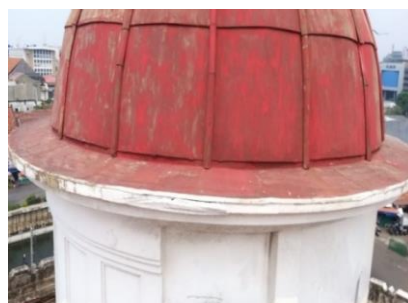
(b) Heritage building roof
