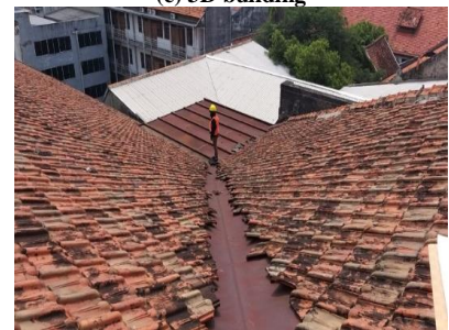
(f) Roof gutters
