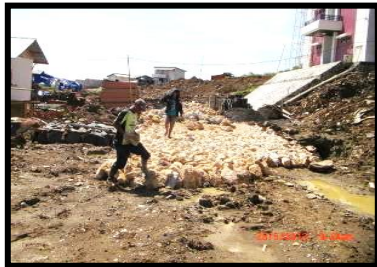
a. Retaining wall implementation
