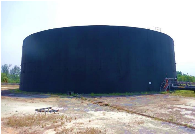
Fig. 2 Storage Tank T105
