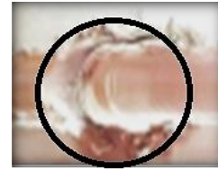
Fig. 3(b) Improper welding and material dragging
